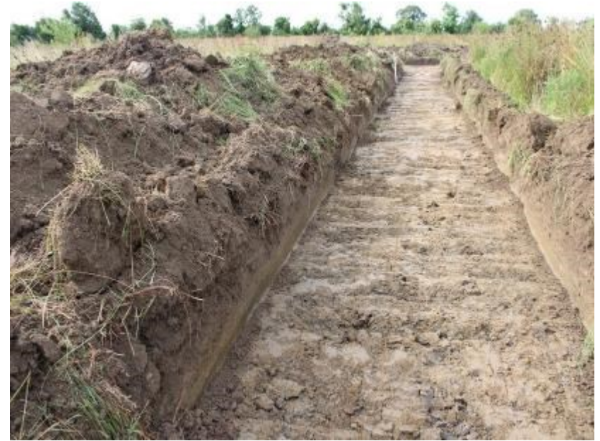
Plate 42: Trench 30 (A), looking NNE
