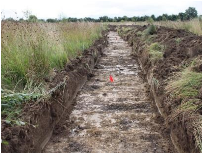
Plate 43: Trench 30 (B) looking NW
